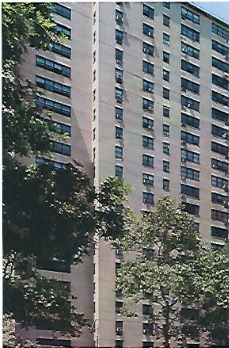
Messaryk Towers, a 1,105-unit Mitchell-Lama cooperative located in the Lower East Side of Manhattan, is working with the City to finance a new boiler plant and cogeneration system and lock-in affordability.
